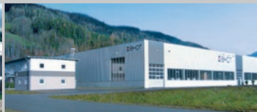
BFT PUMP PRODUCTION AND WELDING CENTER, HOENIGSBERG
