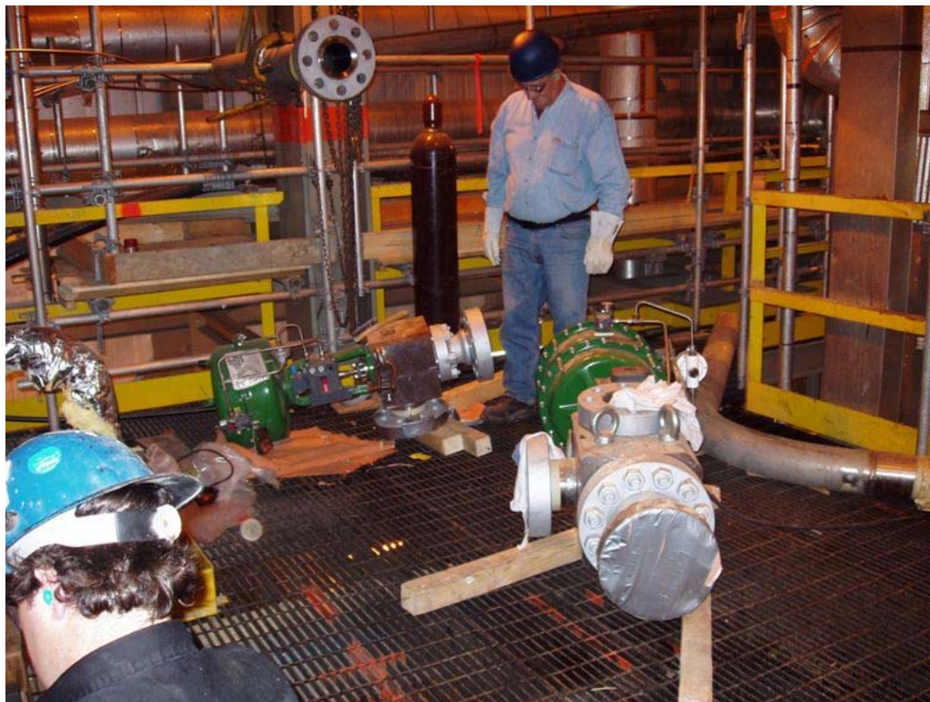
These two large High Pressure control valves going to be installed.
